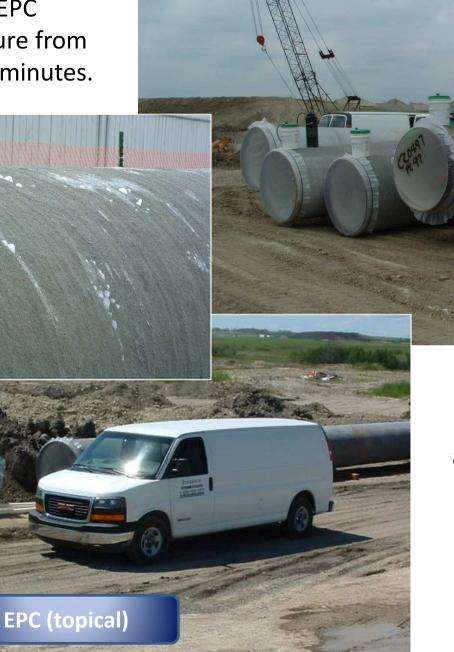
EPC treated surfaces are typically ready for use or handling within 1-hour for pipe or Precast filed parts.
